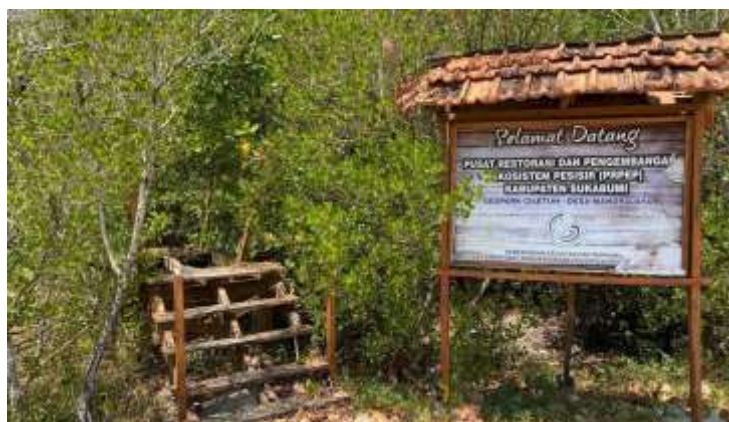
Figure 5. Neglected mangrove bridge reflecting gaps in infrastructure maintenance and local governance, highlighting tensions between development planning and community engagement.
